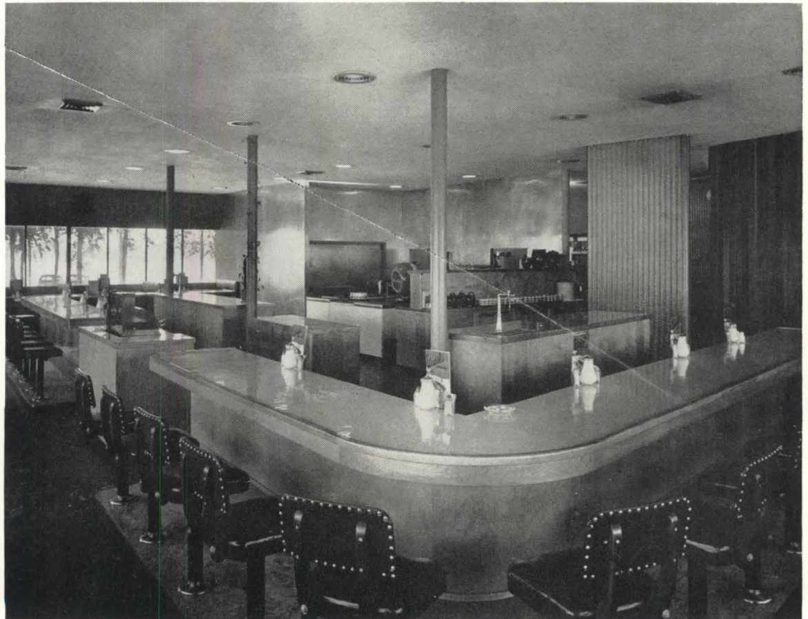
Asphalt tile floor; aluminum walls in service space. Corrugated glass defines the corridor to the toilets.
