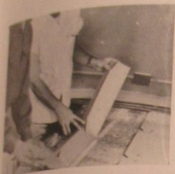
5 Folding the triangle which is the basic structural module of a geodesic dome and geometrically strongest shape for given weight of material.
