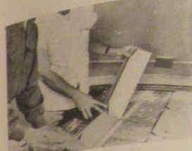
5 Folding the triangle which is the basic structural module of a geodesic dome and geometrically strongest shape for given weight of material.
