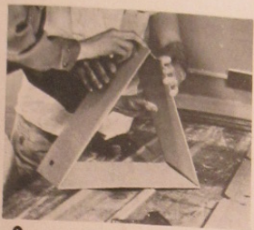
6 Triangles (6) at Tulane were taped but wood dowels will assemble future domes. Domes can be disassembled and shipped flat, or lifted intact.
