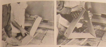
5 Folding the triangle which is the basic structural module of a geodesic dome and geometrically strongest shape for given weight of material.
