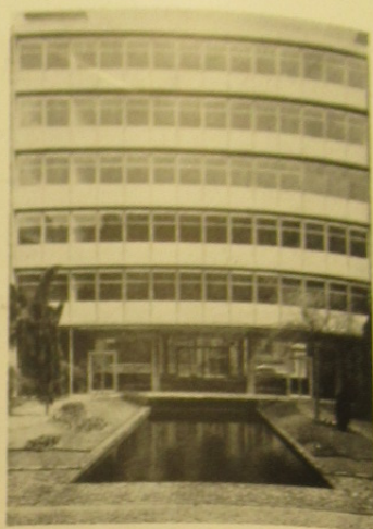
Above: Bauen und Wohnen , No. 6, Munich. Glassed front of Federation Nationale du Batiment, in Paris, made of 126 prefabricated elements. Gravereaux & Lopez accentuated functionalism with Baroque elegance.
