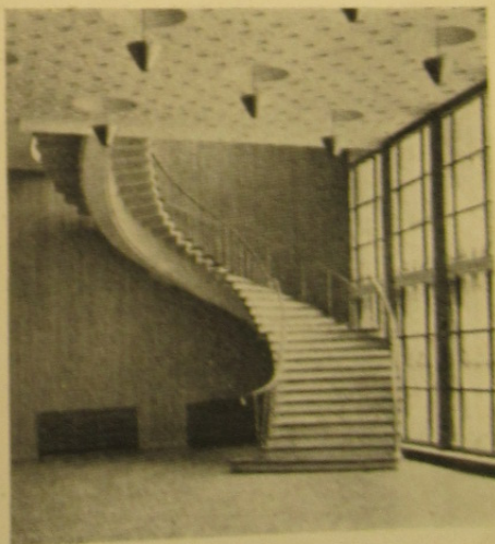
Above: Architektur und Wohnform , No. 4, Stuttgart. Entrance hall of the new Koeln Radio Station building, by P. F. Schneider. Photograph of ground-floor shows suspended staircase—a principle employed throughout the structure to provide better acoustic vibration.
