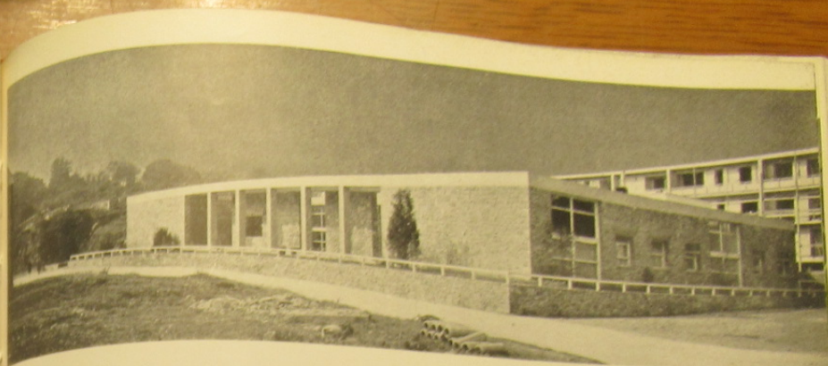
Above and left: the nursery school. Three big windows piercing the heavy walls beyond the colonnade reveal that the heart of this stone block is a sunny play yard. A series of awnings can be used to cast shadows across the yard. Below: the plan. 1 Dressing rooms. 2 Classroom. 3 Playground. 4 Refectory. 5, 6, 7 Kitchens. 8 Bathroom. 9 Personnel. 10 Nursery. 11 Nursing dormitory. 12 Weaned dormitory. 13 Weaned playroom. 14 Disinfection. 15, 16 Staff rooms. 17 Doctor. 18 Isolation. 19 Storage.
