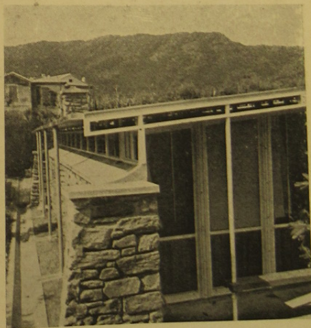
Above: Bauen und Wohnen, No. 4, Munich. A villa on the French Riviera is covered with a thin roof, to soak up the sun, above a regular ceiling. This is the bedroom wing; the living area, in a separate square, is glass-walled.
