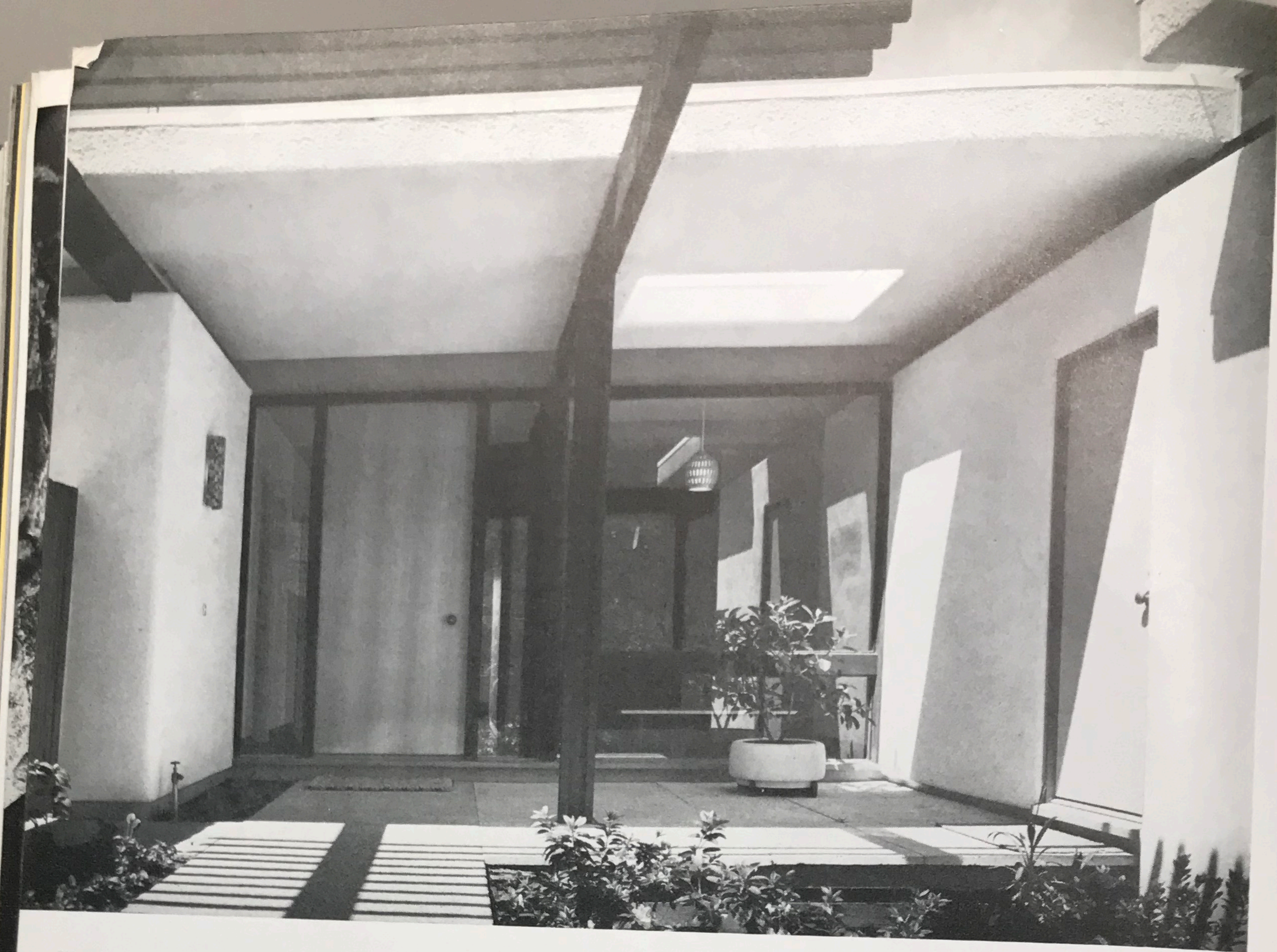
The door in the sunny, open, free entrance way, is solid core with oak veneer which has been varnished in natural. The mosaic wall lamp, by Gruen Lighting, is normally made in a cylinder, which was cut in half to be produced into two half-cylindrical units. They cast a shimmering mixture of beige and green at night.
