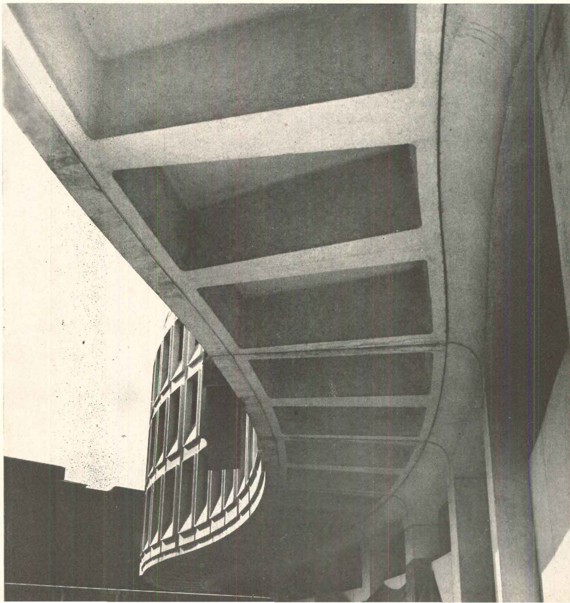
Assembly of the superstructure went from both ends to middle. Cantilever below bears the crucial steel strands.
