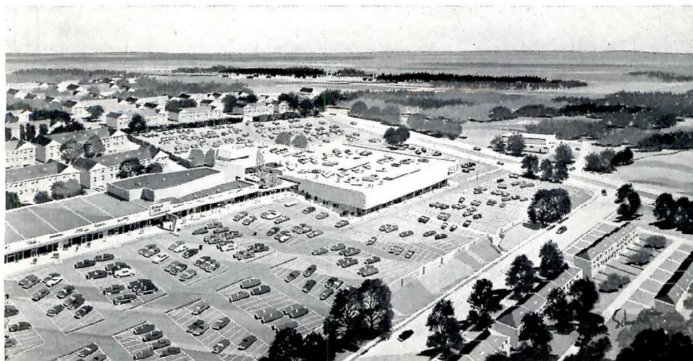
Hecht Co., Northwood Shopping Center, Baltimore, Md.; Abbott, Merkt & Co., Engineers; Daniel Schwartzman, Architect
