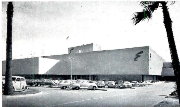
Emporium, Stonestown, Calif.; Welton Becket & Associates, Archts.
