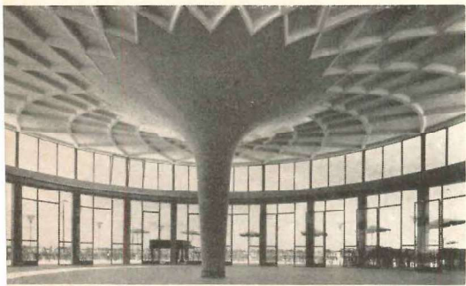
A highly expressive geometric pattern was formed in the ceiling of this restaurant designed by A. La Padula through a refinement inervi's pre-fabrication techniques. Precast, coffered sections, about 1-in. thick were assembled on a platform with spaces left between for reinforcing of the stiffening ribs
